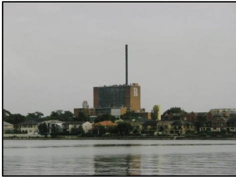
Figure 19. View of subject site from Hen and Chicken Bay, c. 2007. 39
