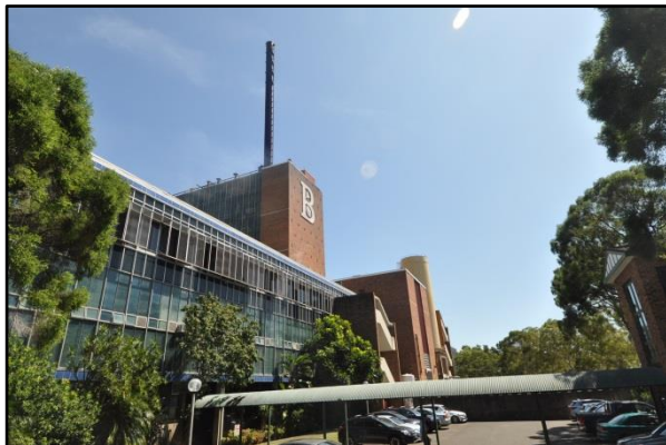
Figure 23. View of the covered walkway joining the eastern façade of the factory to the administration building.
