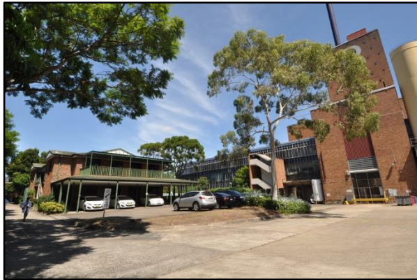
Figure 27. View south-west encompassing the northern facade of the administration building and a detail of the eastern façade of the factory.
