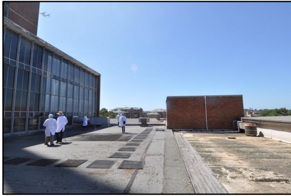
Figure 37. Roof space located on second floor.
