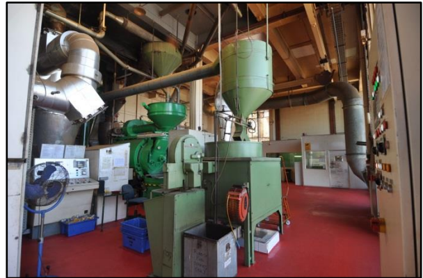
Figure 36. Detail of space located on the second floor.
