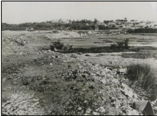
Figure 9. Reclamation works at Exile Bay, c.1930. 15
