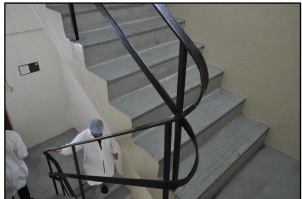
Figure 42. Curved steel handrails located in stairwell located between floor five and floor three.
