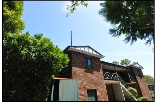
Figure 26. Eastern façade of administration building with half-timbered gables shown.
