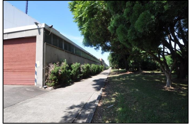
Figure 32. Western façade of the factory with landscaped area located along the western boundary evident on the right.
